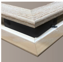
MITER ALIGNMENT KEY INSTALLED
